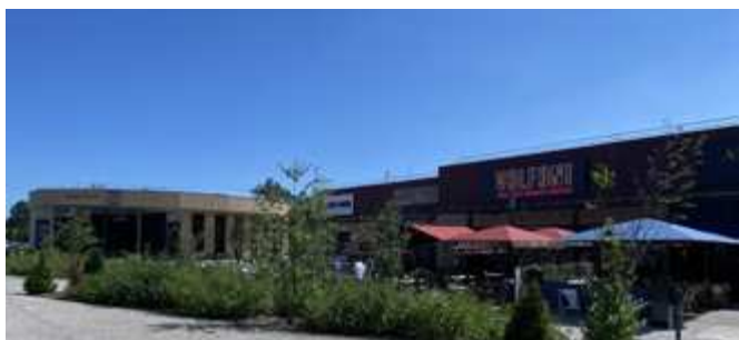
Chamblyrama - Facade restaurant Volfoni
