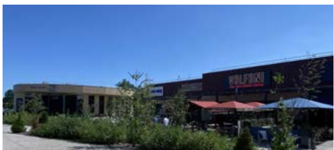
Chamblyrama - Facade restaurant Volfoni
