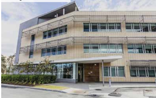
Building 8 – Dublin – Irlande
