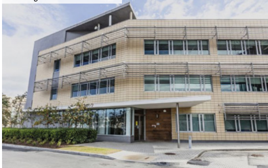
Building 8 – Dublin – Irlande
