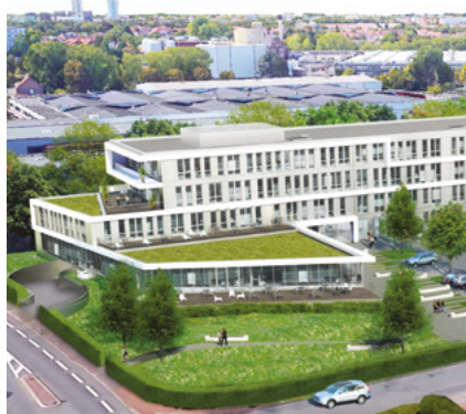
Business Office – bât. A – Marcq-en-Barœuil (59)
