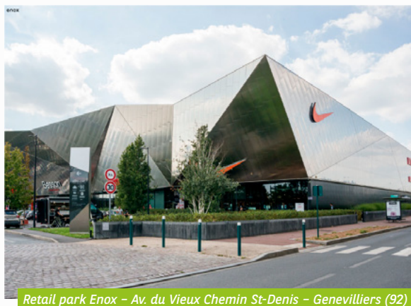
Retail park Enox - Av. du Vieux Chemin St-Denis - Genevilliers (92)
